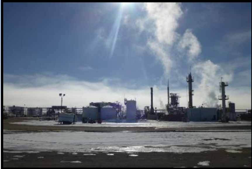
Foreland oil refinery, Railroad Valley, Nye County
